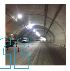
The Riva tunnel is a 562 m (1844 ft) long four-lane motorway tunnel located northeast of Istanbul, Turkey. The tunnel's excavation span is 22 m (72 ft), while the final lining diameter is 18 m (59 ft). This makes it one of Europe's biggest tunnel cross sections.
