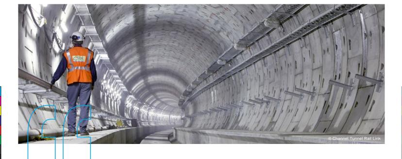
The final component of the celebrated high-speed rail line connecting London and Paris, the Channel Tunnel Rail Link (CTRL) included more than 25 miles (40km) of precast-lined tunnels in water-bearing sands and London clay, with water pressures up to 3 bar. Contracts 220 and 240 specified a steel fiber reinforced segmental lining to ensure corrosion resistance, structural performance and a more efficient production process.
